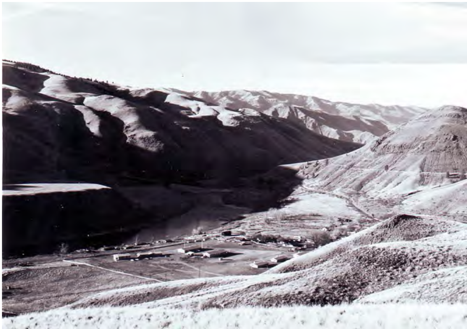
Slate Creek Ranger Station, 1962 Courtesy of U.S. Forest Service.
