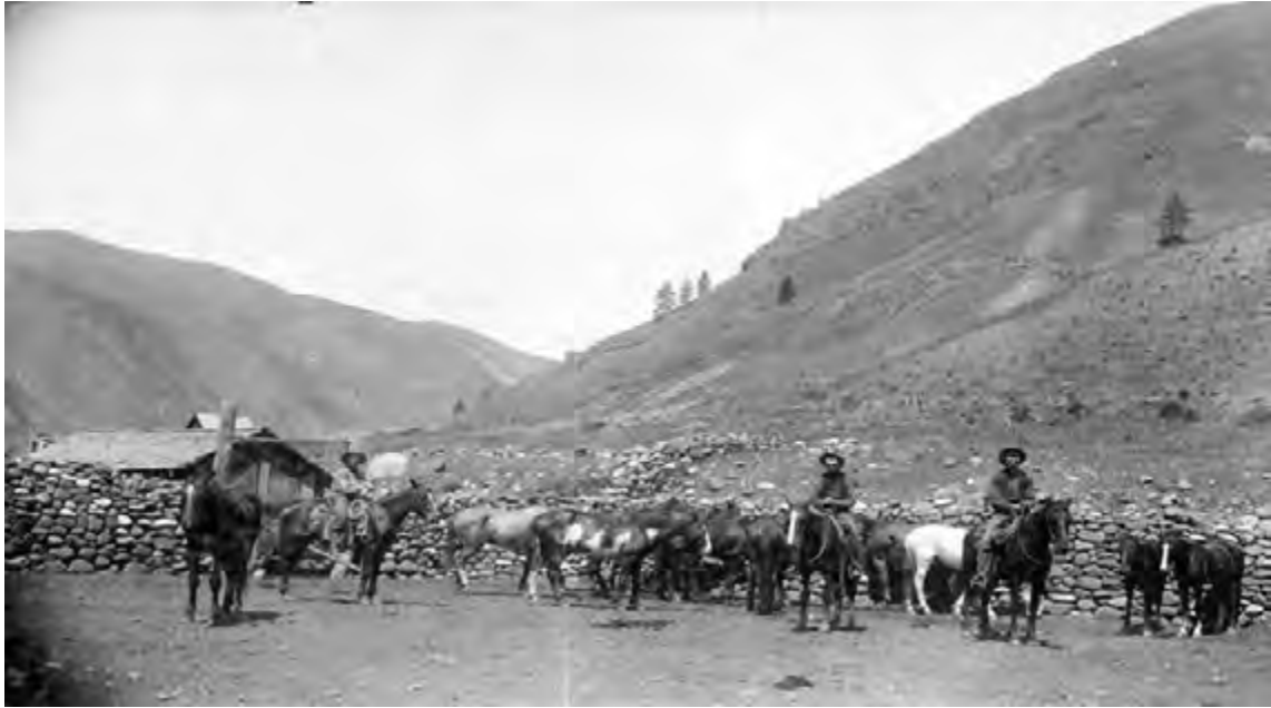
Freedom (Slate Creek) Post Office in the far left behind rock wall. Courtesy of Idaho Historical Society. Copyrighted by the Idaho Historical Society.
